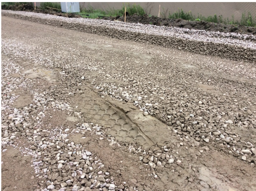
Figure 7.7 Condition of 9-inch deep large stone subbase section after first construction iteration.
