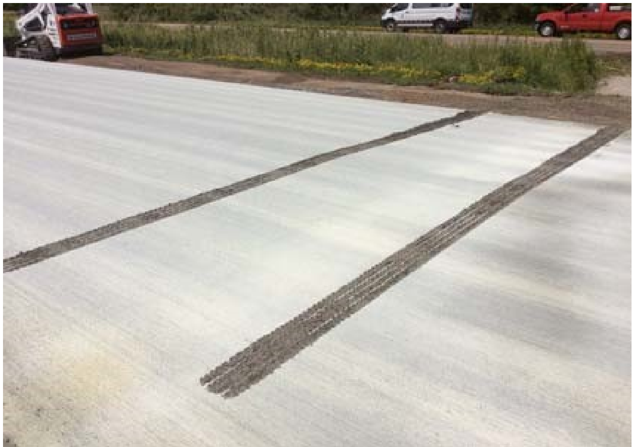
Figure 5.6 Rut depth ranged from 0.25 inch in the outside lane to 1.5 inches at the edge of inside lane.
