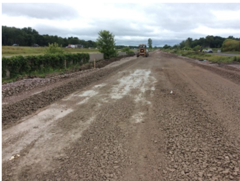
Figure 7.8 Comparison of large stone subbase condition: 9-inch thick Cell 128 (foreground) and 18-inch thick Cell 227 (background).
