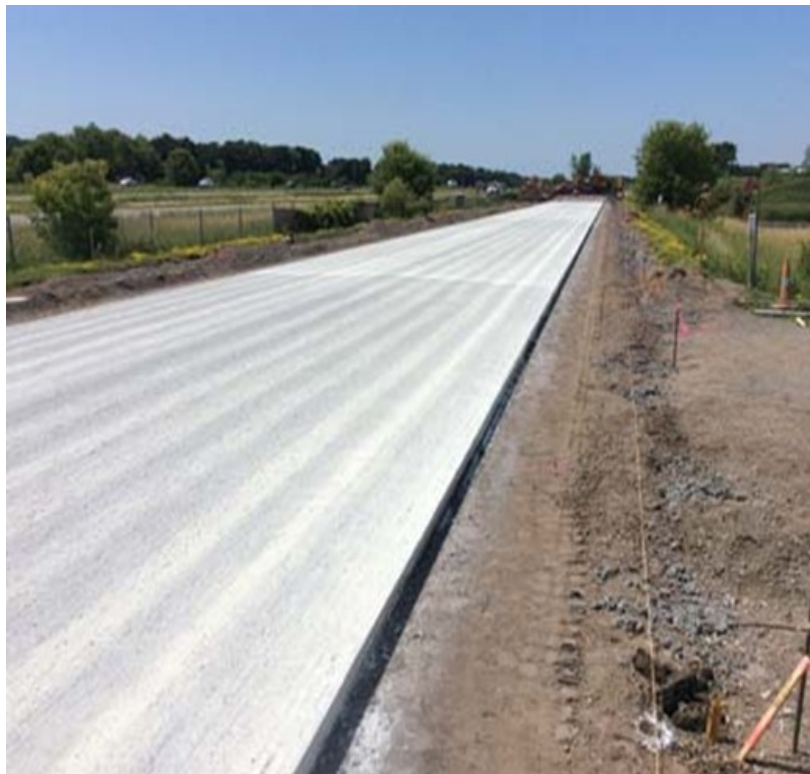
Figure 5.4 Panoramic view of Cells 124 to 624 pavement after placement and application of curing compound.
