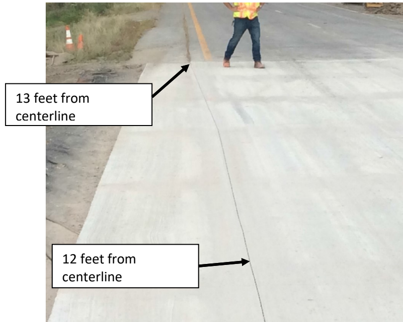
Figure 4.11 Inadvertent longitudinal sawcut misplacement in FRC Cells 705 and 805.
