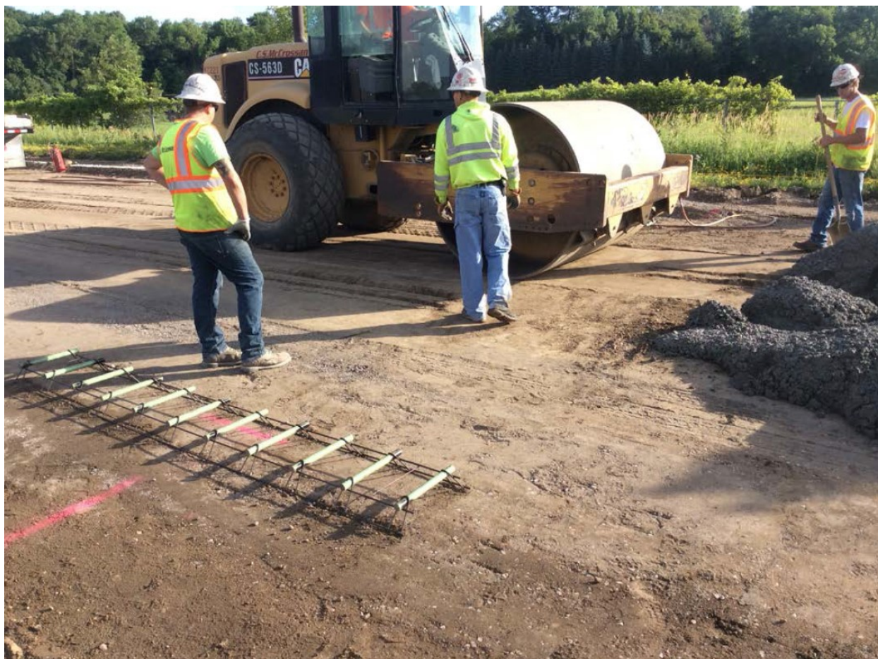
Figure 6.4 Contractor shaping aggregate base in front of paver with drum roller, Cell 238.
